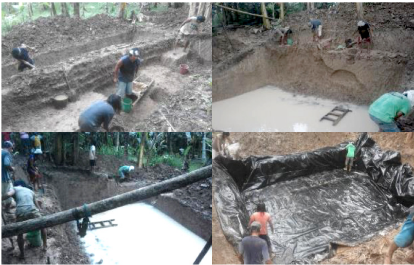
Figure 3. Construction of the water impounding system.
