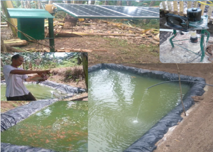
Figure 8. The Constructed Irrigation System
