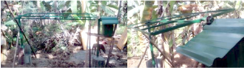
Figure 4. The Constructed Solar Panel Mount
